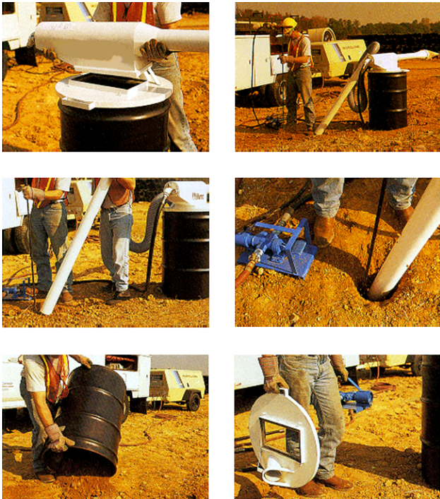
Vacuum Excavation Method
